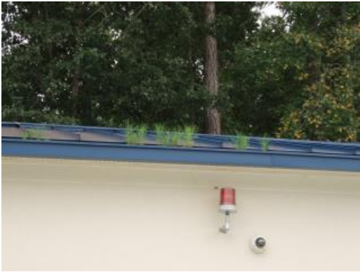
Gutter at Lazy River Pump Room
