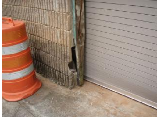
Repair CMU Wall
