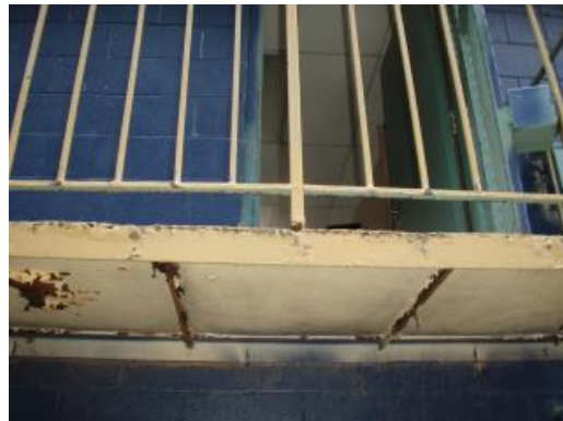
Replace Metal Stairs Located Rear of Building
