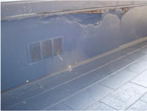
Soffit at Rear of Building
