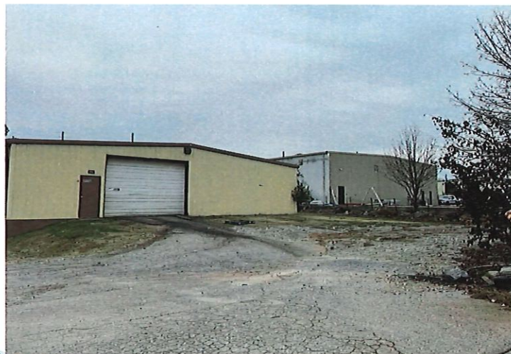
VIEW FROM SSML ROAD OF ALLEN 2825 SSML RD & VARIABLE STEEL BUILDINGS
