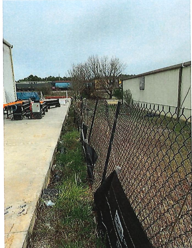
Figure 7: Existing fence on southside of building
